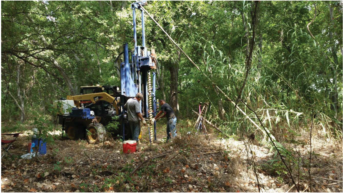
Photo 3 – View looking at Boring 3 drilling operations.
