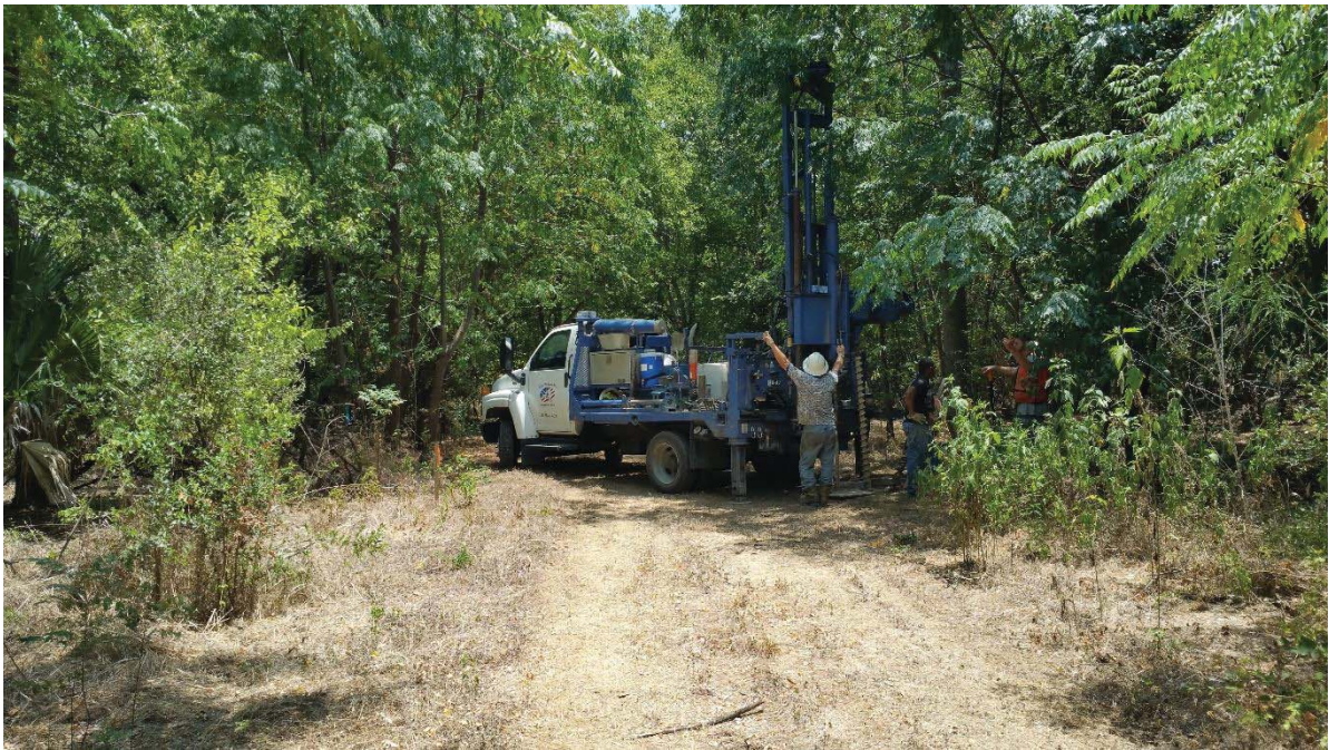
Photo 1 – View looking at Boring 1 drilling operations.
