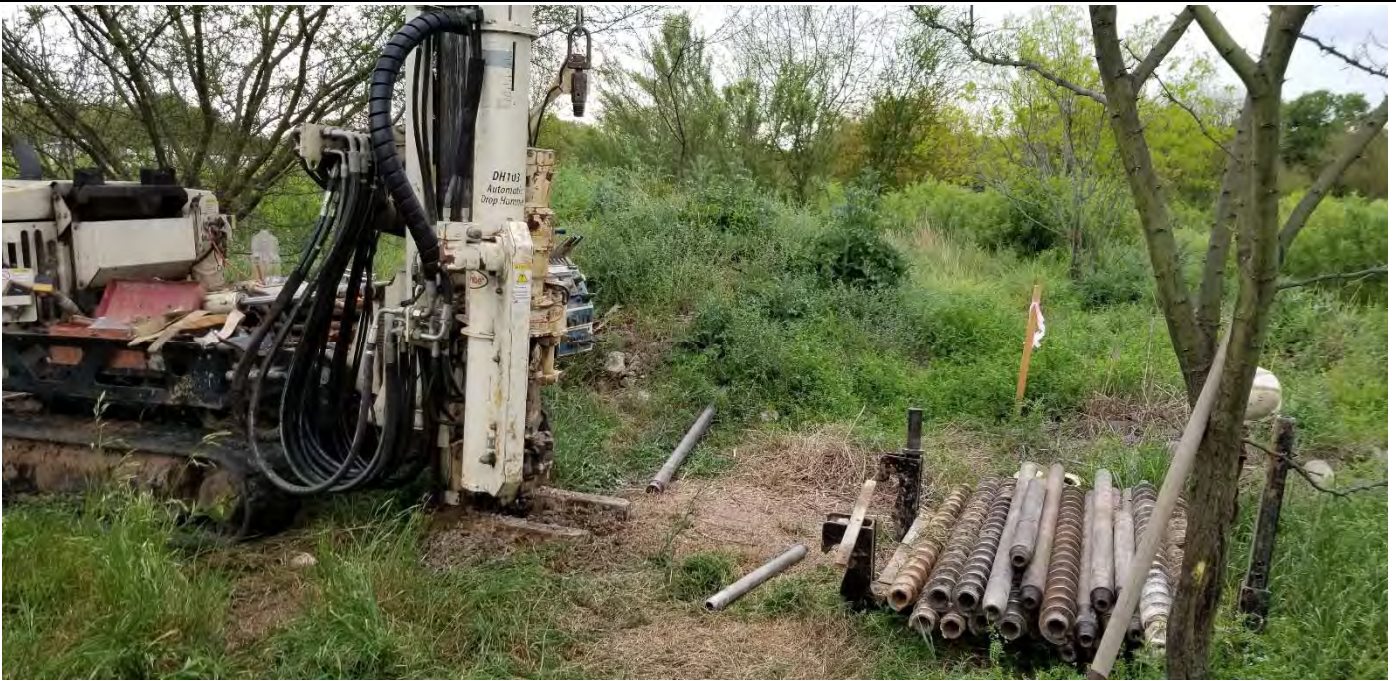
Photo 1 – View looking at Boring 4 drilling operations.
