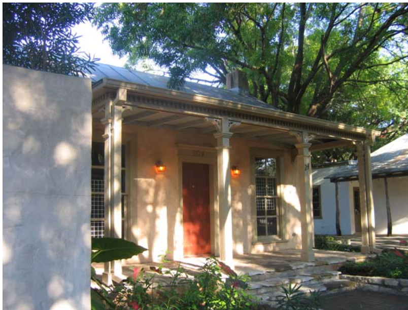
Building 24 at La Villita is marked on the porch but also has reference to the number 101 above the doorway
