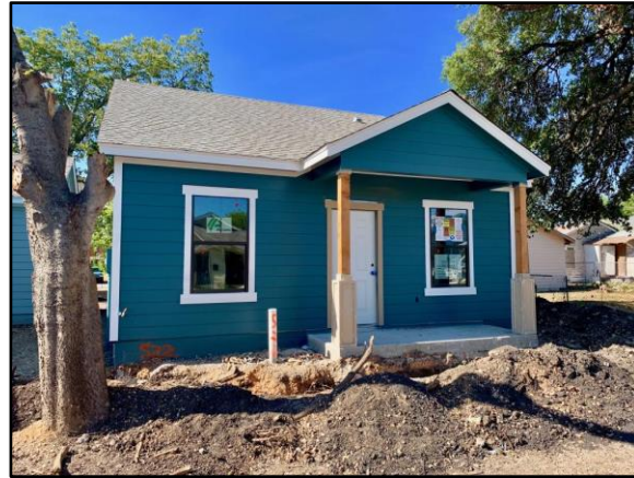
White shingles, or "cool" roofs, are encouraged to reduce heat gain and improve energy efficiency.
